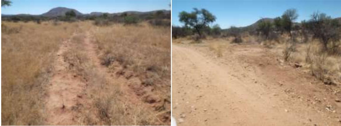
**Figure 4a,b. Road drains: On the left is a long, narrow angled drain blasting water at the landscape below. On the right is a short, flat drain that spills water calmly.**
