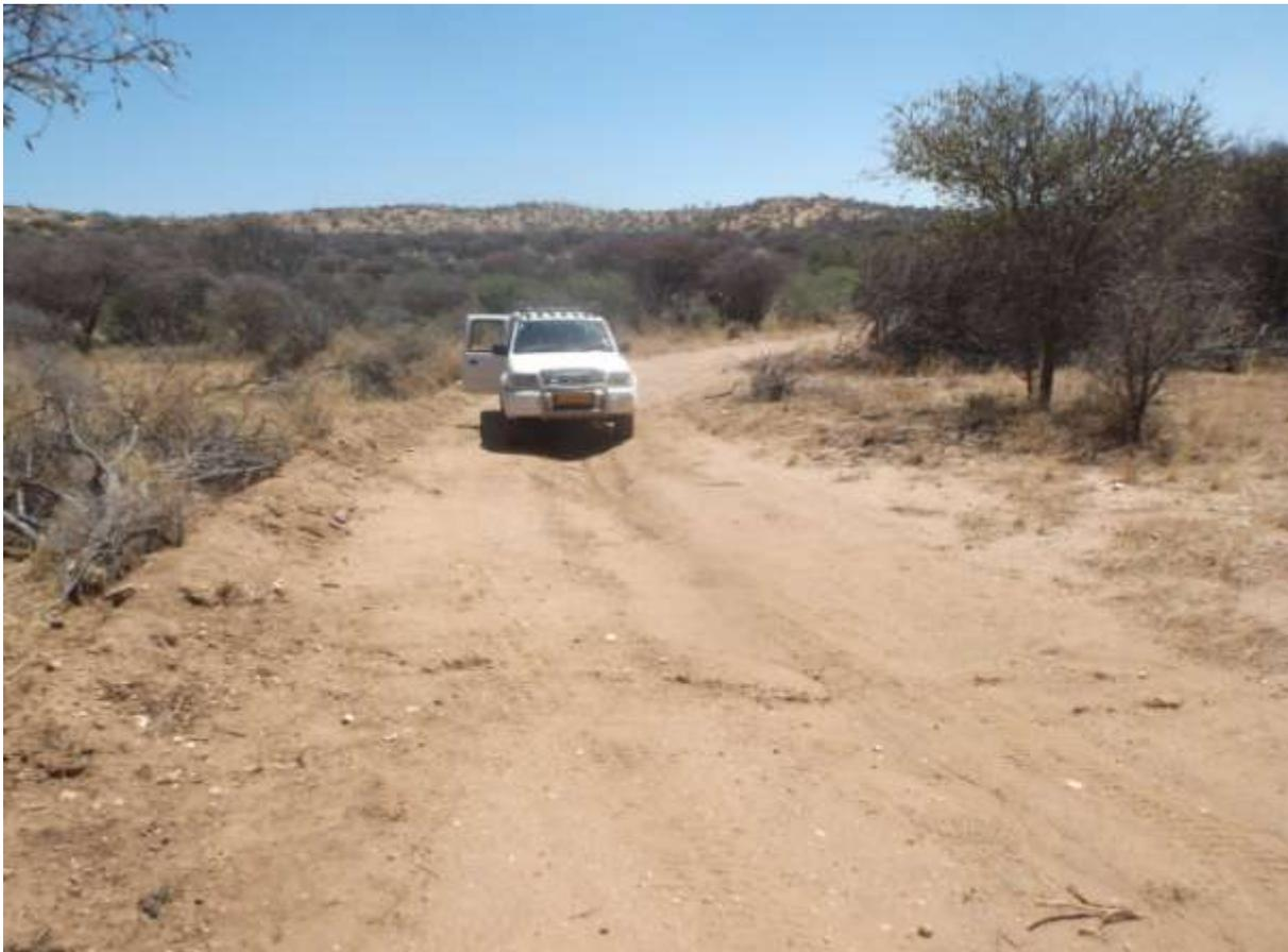
Figure 5. A “road creek” with a windrow on the down slope side (left) that keeps the water on the road to discharge violently when it finally breaches the windrow.
