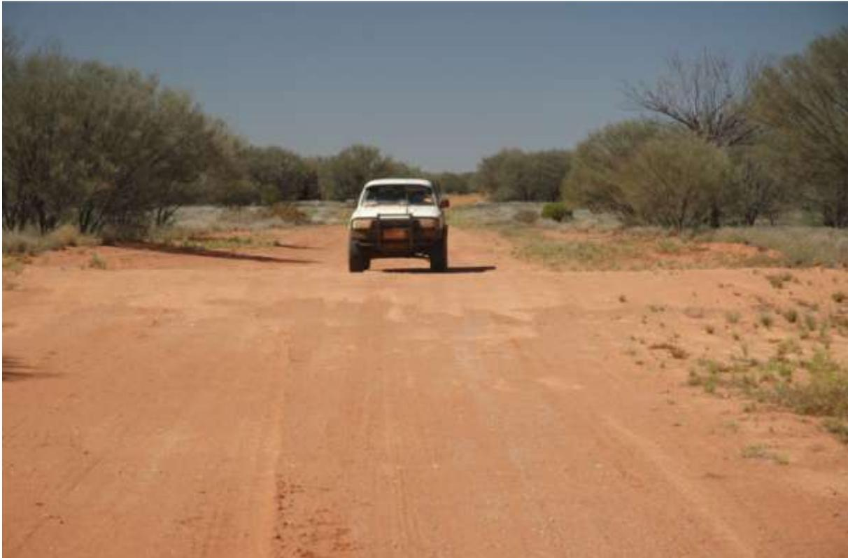
**Figure 3. This farm road was a virtual river flowing towards the reader, with channels and sand deposits along it. Now it is smoothed out and has trafficable bunds to spill any harvested water calmly back onto its natural course. This is sandy country, so some material was brought in for the bund from nearby. This road has had major storms over it with no maintenance required at all.**
